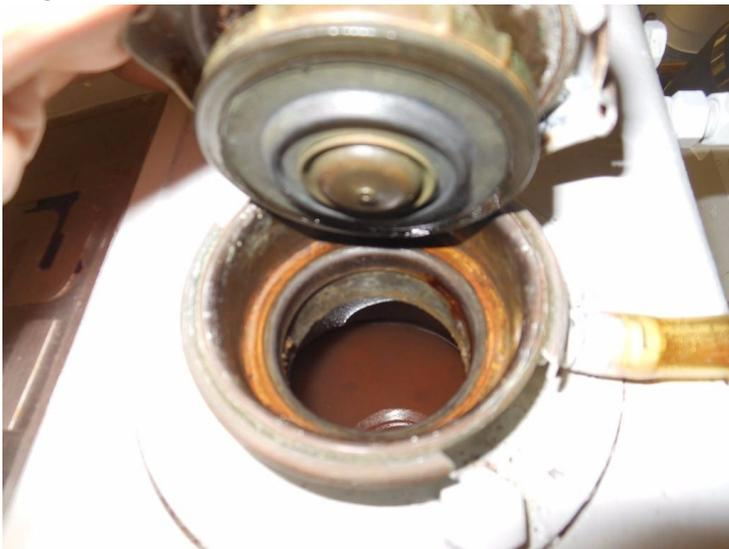
**Because they must maintain an air void within when not used with a recovery bottle, steel and cast iron expansion tanks are prone to rusting.**
