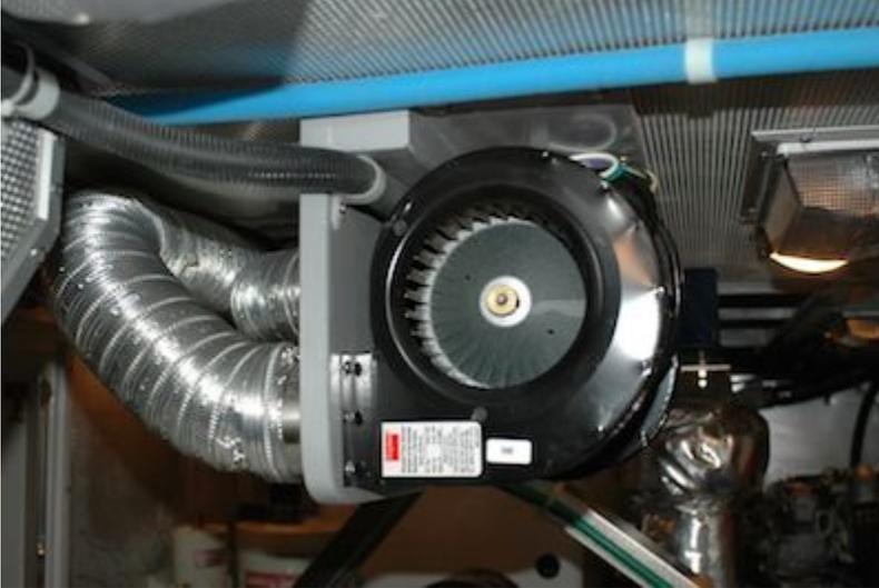
All but the smallest engine and engine room installations will almost certainly require forced ventilation. Fans must be rated for continuous duty, like the “squirrel cage” model shown here.
